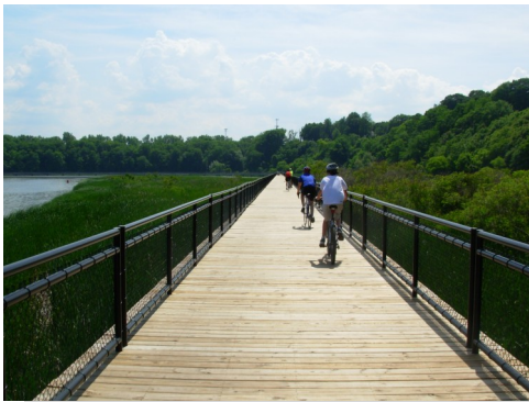
Riding on the footbridge at Turning Point Park
